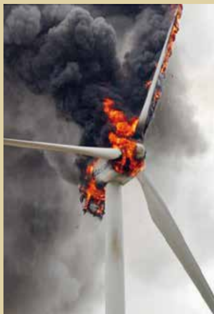
Slika 5: Požar na vetrni elektrarni ( http://taproot.com/common-wind-turbine-equipment-failure-modes/ )
